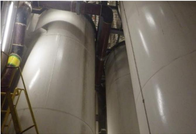
The four cement silos were well located in the Port fwd column were satisfactory with all surfaces and pipe work valves corrosion free. Good access was possible at both upper and lower portions of the silos.
