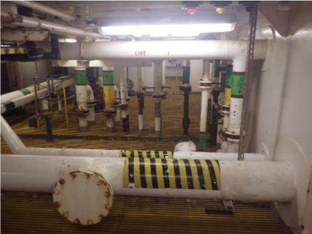
The mud tanks were empty during the survey condition, well cleaned out and in a satisfactory visual condition. No corrosion was noted on tank surfaces (viewed from above)
