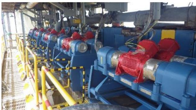
The five shakers were seen to be freshly painted and were in a satisfactory condition. All associated manual valves were found to be free to operate and the whole system free of any serious corrosion.
