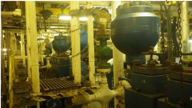
Mud pump discharge manifold view
