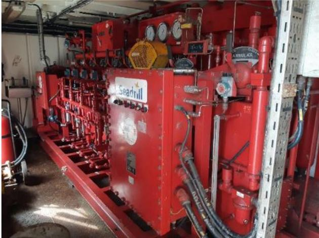
The BOP / Diverter accumulator unit.
