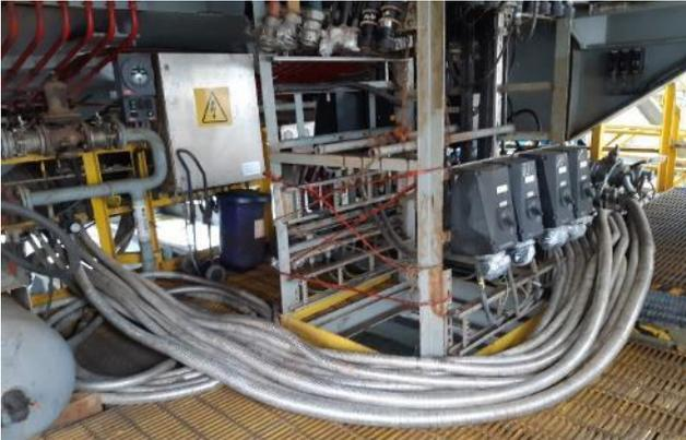
The BOP control hoses still connected to the control unit and stored under the BOP accumulator unit.
