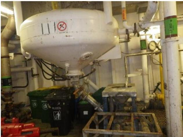
Both surge tanks were in a satisfactory condition, well painted with no signs of corrosion. The surfaces were undamaged and free of hammering marks.
