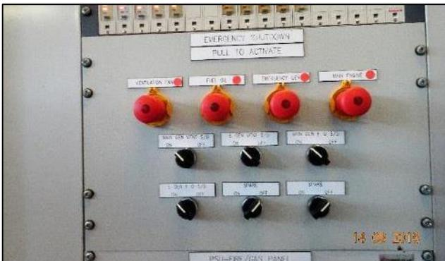
C.1.6 ESD panel in ballast control room (Included within the fire & gas rack enclosure)
