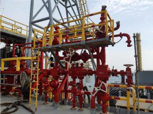
The Standpipe and Cement manifolds mounted on the package which made up the drill floor.
