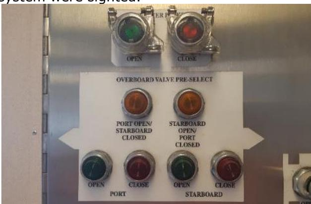
The diverter controls on the BOP control panel in the Toolpushers office.
