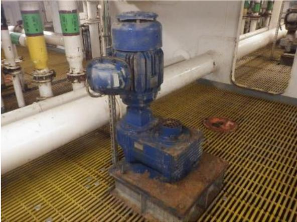
None of the sixteen (16) agitators installed were in use during the survey and were in a fair condition during the survey however the corrosion issue's seen on all of the mud pit agitators should be addressed before becoming a serious problem.
