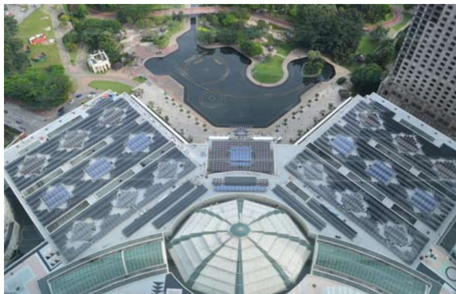
■ Aerial view of Solar Photovoltaic panels on the rooftop of Suria KLCC
