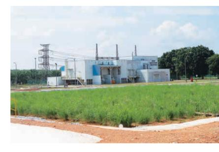
Developed within a two-acre piece of land, the reed bed wastewater treatment system uses wetland vegetation and microorganisms to reduce the concentration of pollutants in the wastewater. The microorganisms in this system breaks down, remove and transforms hazardous contaminants into less toxic forms. The reed plants, meanwhile, play a significant role in creating an aerobic environment which is required for microorganisms to thrive.
