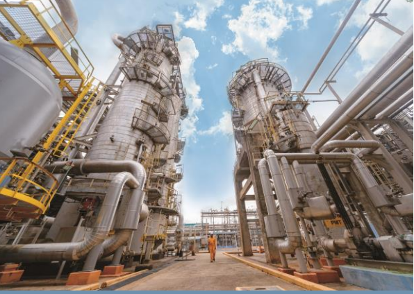
Uninterrupted gas supply
