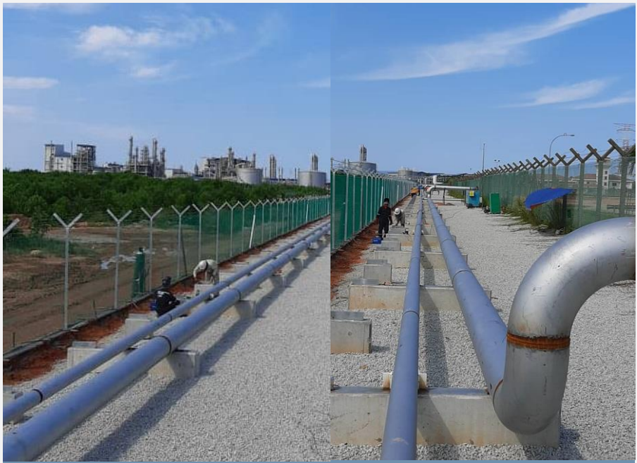
Piping construction for steam supply to Polyplastics Asia Pacific Sdn Bhd
