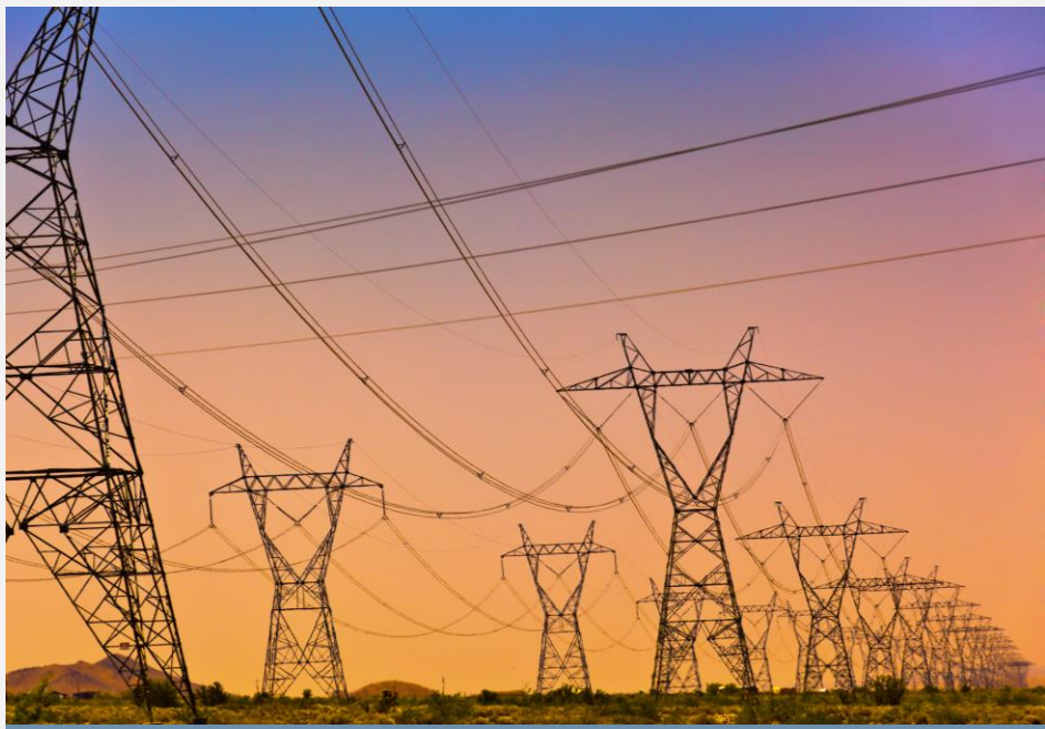
Secured electricity supply to Kaneka (Malaysia) Sdn Bhd
