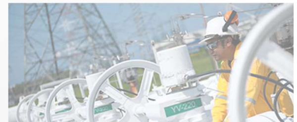
42km Lateral Gas Pipeline to Pulau Indah
