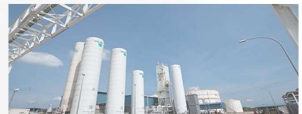
Oxygen Backup Facility
