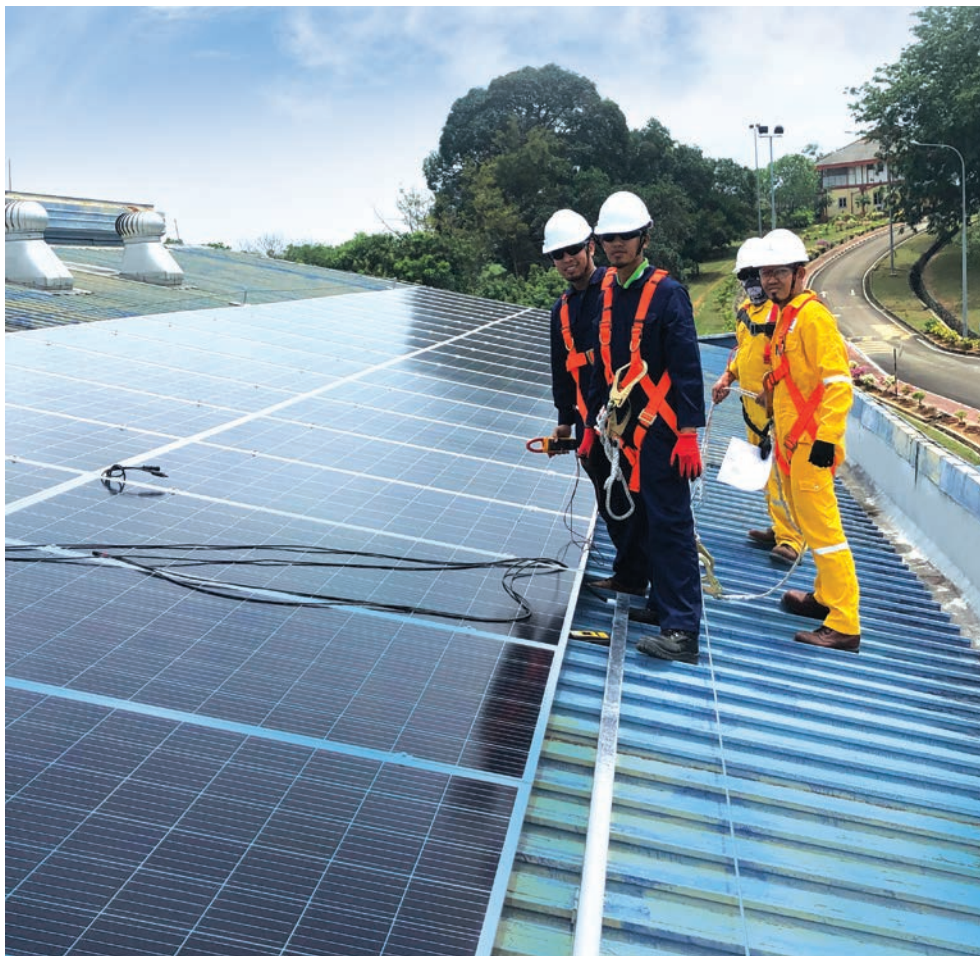
Solar PV system installed at PGB Seremban Regional Office rooftops
