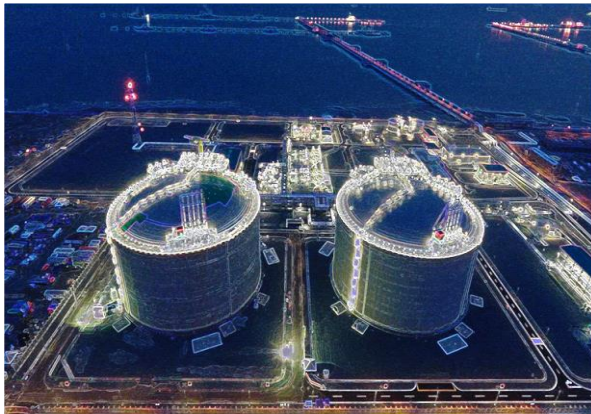
Two LNG storage tank with storage capacity of 200,000 m 3 each
