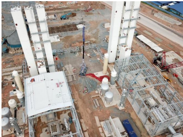
Train 1 & 2 to separate atmospheric air into oxygen and nitrogen
