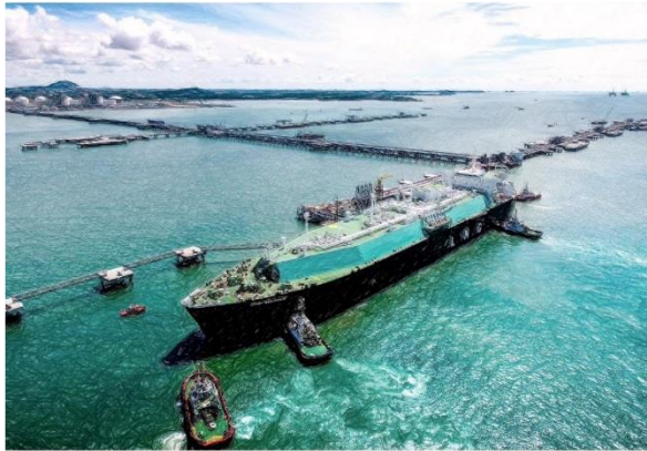
Jetty able to receive LNG carriers up to 260,000 m 3 for unloading and reloading
