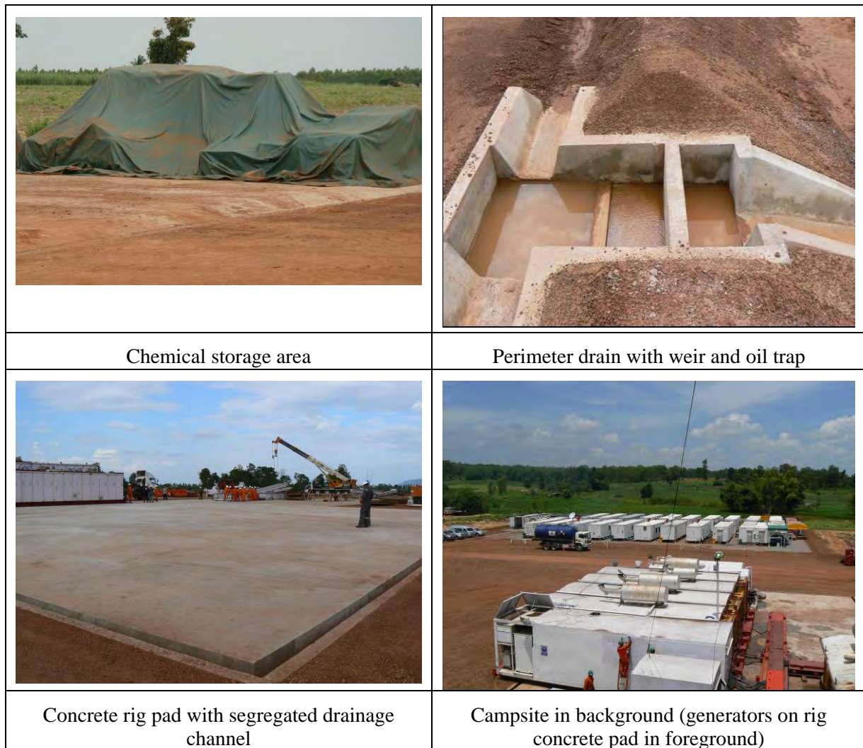
Figure 2-27: Photos of a Typical Exploration Drilling Well Site and Facilities
