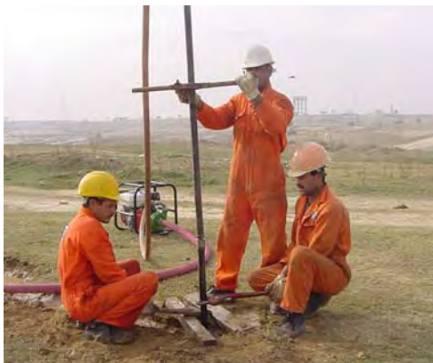
Figure 2-15: Examples of Shot Hole Drilling
