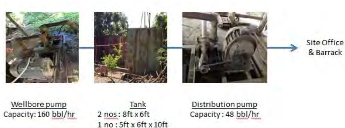
Figure 2-50: Existing Water Utility System
