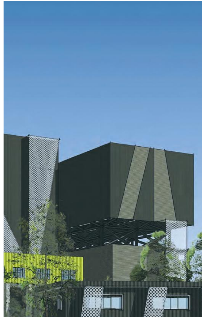
Figure 7: Incinerator by Cypark Resources Bhd
