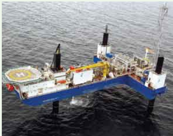
PETRONAS' oil producing operations at Block 1, Turkmenistan
