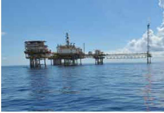
The Erb West platform located offshore Sabah
