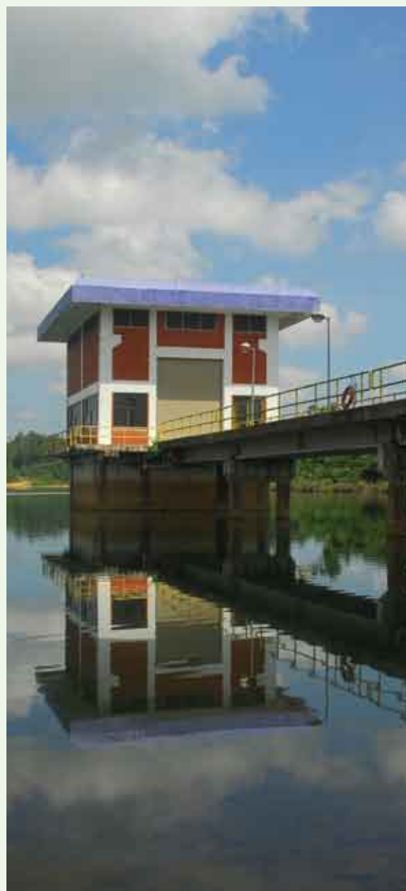
The Draw-off Tower near the off-river storage area at BAKIPC
