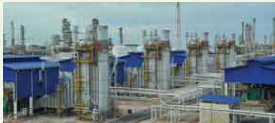
A cogeneration unit located at PP(M)SB
